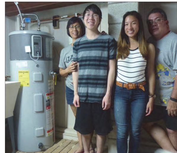
The GE Geospring® model pictured here with one of our pilot families has various operating modes that offer different levels of efficiency and can be controlled remotely via the web or smart phone application by addition of the GE Connect Plus module.
