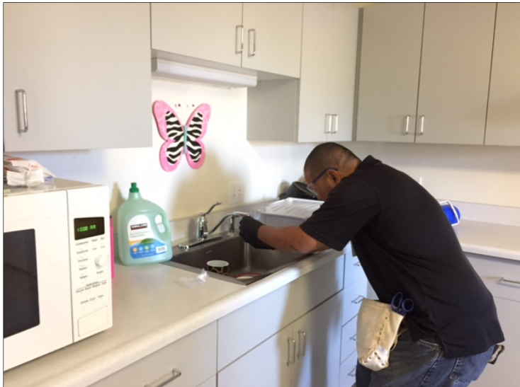
A Hawai'i Energy technician installs a faucet aerator at a property participating in the Energy Smart 4 Homes program. These measures are an important portion of the ES4H package, helping residents to reduce both energy and water usage.
