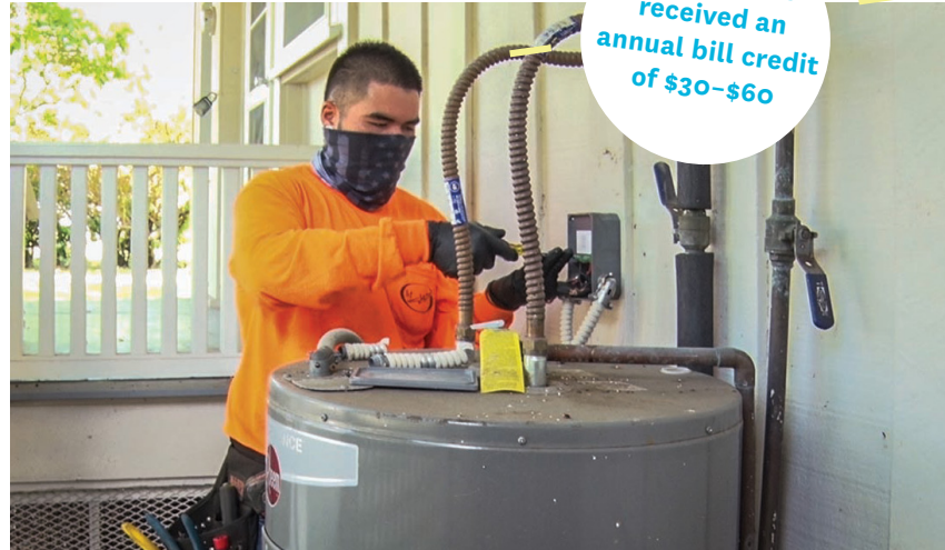
M. Watanabe electrician in Hau'ula installing Shifted Energy 's Tempo device on a home's water heater
